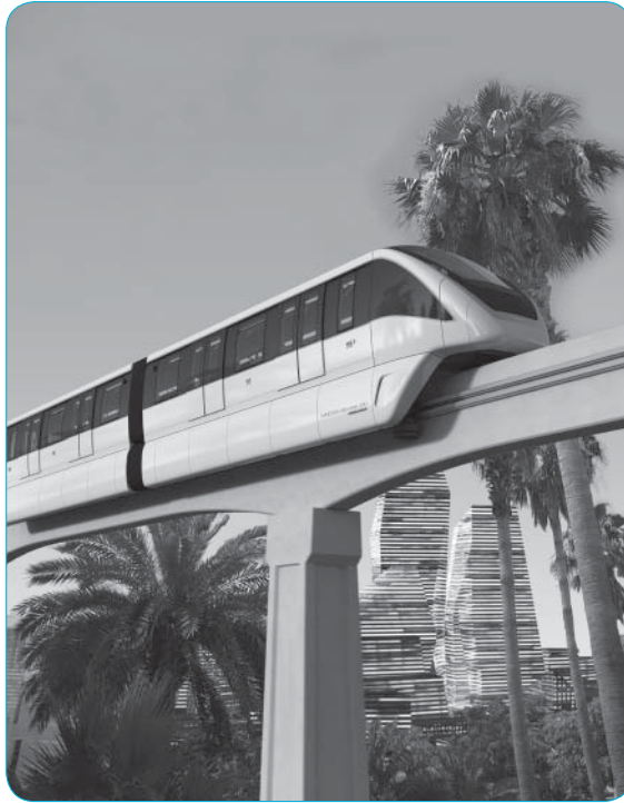
FIGURE 1 On May 31, 2010, Bombardier announced that it had been awarded the contract to Design, Build, Operate, and Maintain (DBOM) a transportation system for the King Abdullah Financial District (KAJD) in Saudi Arabia. Bombardier will be implementing a version of its fully automated BOMBARDIER INNOVIA Monorail 300 system. [© Bombardier Inc. or its subsidiaries. All rights reserved.]
