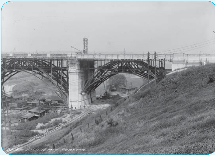
FIGURE 1 The Prince Edward Viaduct under construction. The lower level, eventually used for a subway, can be seen below the top level road. (Photograph reproduced with permission: City of Toronto Archives, Series 372, Sub-Series 10, Item 840.)
